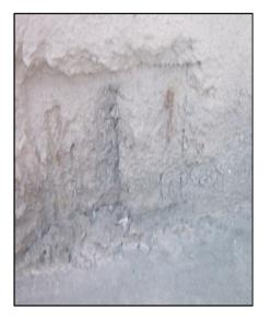
• Honey combing and exposed steel reinforcement/dowels noted in connected patch of ducting connection area.
