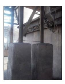
• The pipe rack i.e. vertical members, horizontal members, cross bracings and M.S sheets etc. noted with corrosion and peeling of paint due to the environmental effects.
