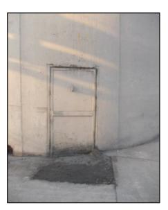
• Unfinished patches noted on the external periphery of the chimney, at few locations, which might made to fix anchor fasteners.
