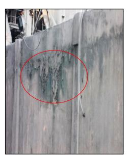
Unfinished through holes are made in masonry walls to pass the electrical cables from external sides; it might be the source of leakage. Please refer photograph below.
